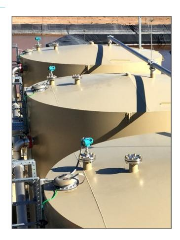
HAWK was able to install a CGR 2-Wire Hart device within 2 weeks to prove the ease of set-up and commissioning and a finished CGR MODBUS version within 6 weeks of the request. Oil level and Salt Water Level accuracy compared with hand dips done over a 3 day period with very good results and the customer's reaction was "WOW".
