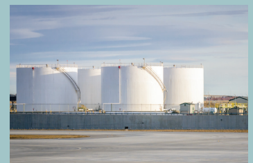
Tank to Tank
